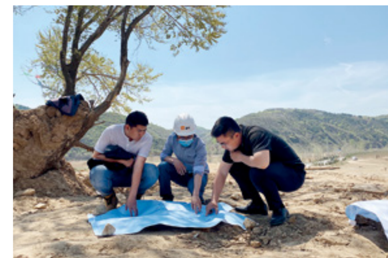
▲ Wang Jia (first from right) discusses about the drawing for Mafang Theatre with his team members Yan Huan and Wang Tao at the construction site to make sure that the construction on site could run smoothly.
