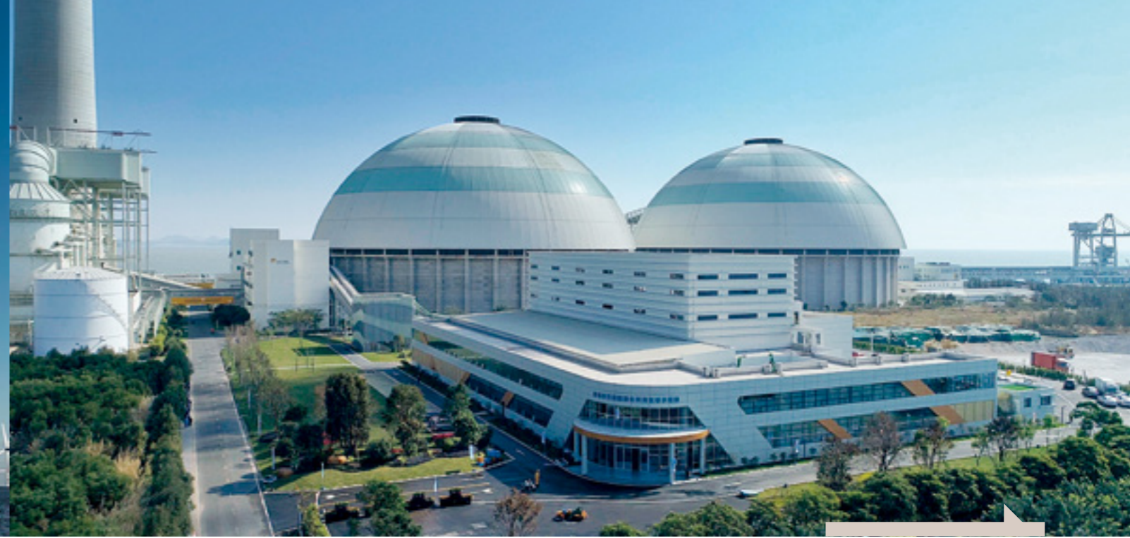
CR Power's Haifeng Power Plant Sludge-Coupling Mixture Project
