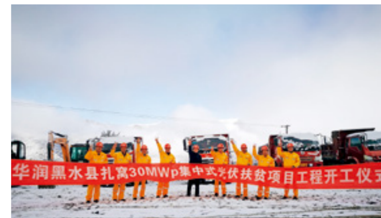
▲ On April 1 st , 2018, CR Power’s 30MW Photovoltaic Project for Poverty Alleviation in Zhawo Township, Heishui County officially started in ice and snow.
