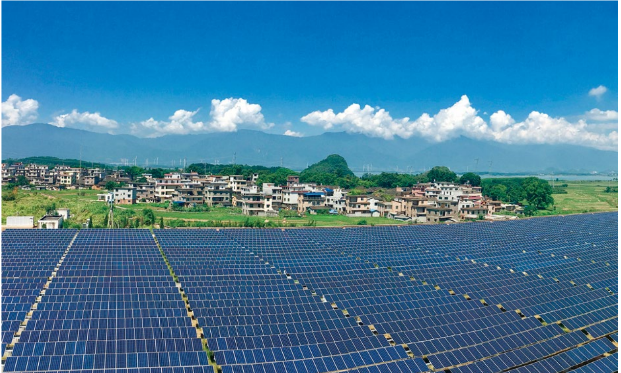
^ The 6MW Photovoltaic project in the Circular Economy Industries Demonstration Zone in Hezhou was the first of this type invested by CR Power in Guangxi, and the total investment was around 44 million yuan. When completed, it would supply 6000MWh clean power to the region, working as an import part of the complementary energy mix consisting of wind, solar, and thermal power in the Demonstration Zone.
