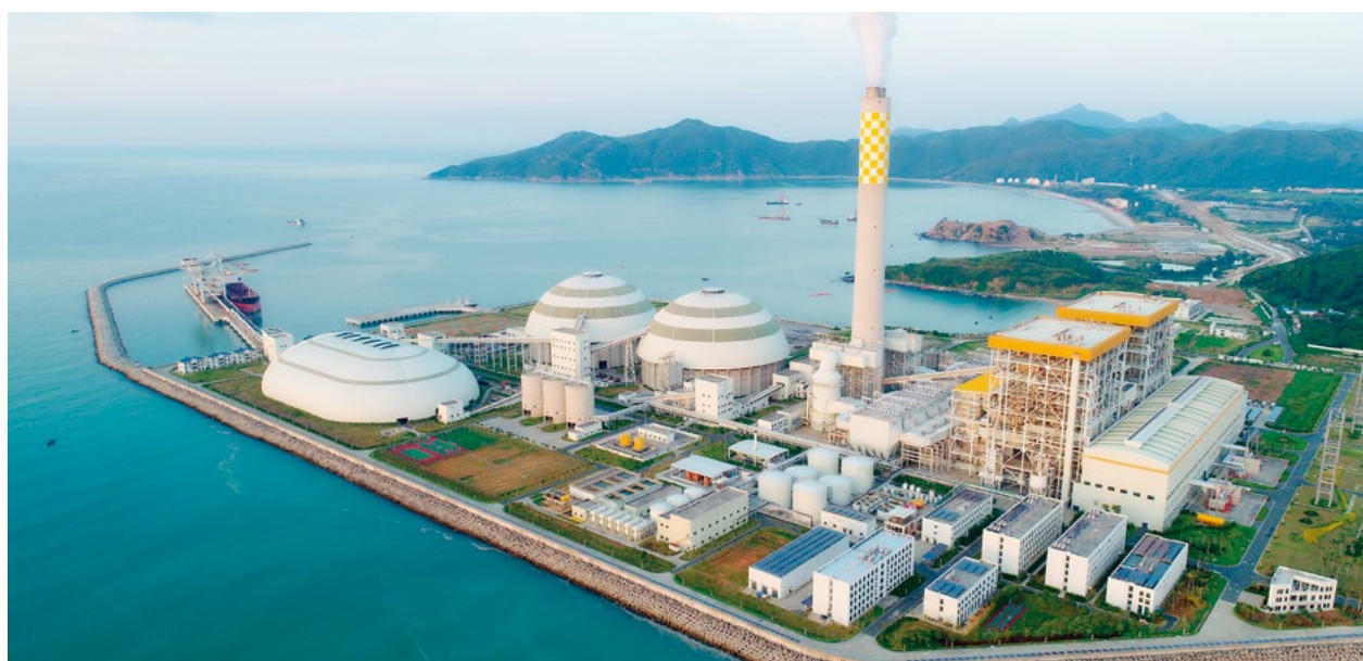
▲ The Carbon capture test platform of CR Power Haifeng Power Plant is one of the 3 major medium-scale test bases for Carbon capture technology in the world.
