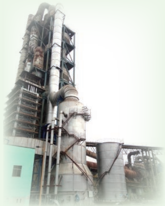
The 3# desulfurization system of China Resources Cement (Changjiang) Limited
