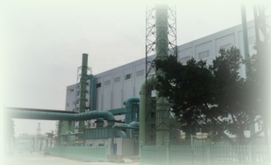
The demonstration project of urban waste co-processing of China Resources Environmental Protection Engineering (Binyang) Company Limited with a handling capacity of 300 tons per day
